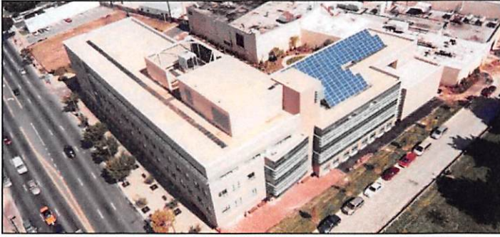
Takoma Park/Silver Spring Health Science Building Photovoltaic Array
