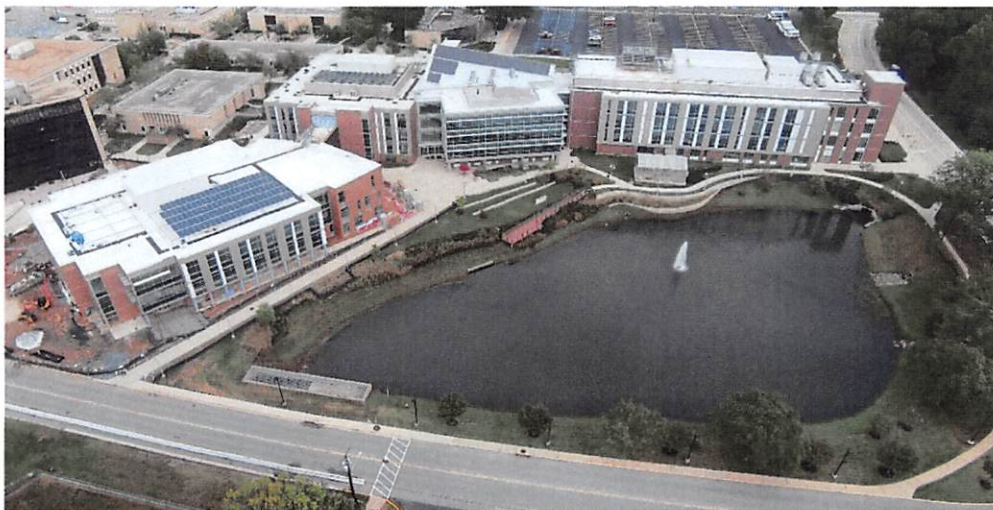
Science Center (SC) on the Rockville Campus (top right) Science East (SE) middle LEED Gold Certified, and Science Center West (SW) LEED Silver Targeted bottom left Opened January 2017
