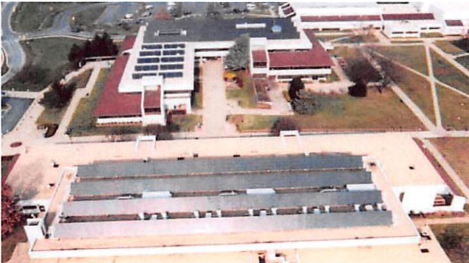
Germantown Campus Photovoltaic and Thermal Arrays
