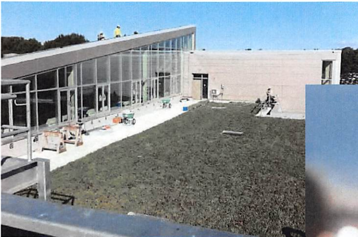
Green Roof and Daylight Atrium Rockville Campus
