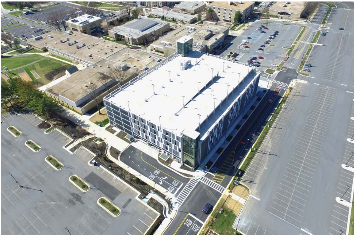
Rockville North Campus Garage (2017)
