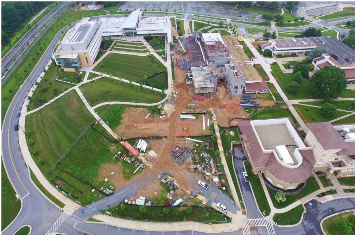
Germantown Science and Applied Studies Renovation Phase 1 (June 2018)
